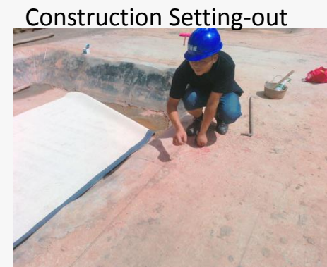
Large-scale Membrane Paving
